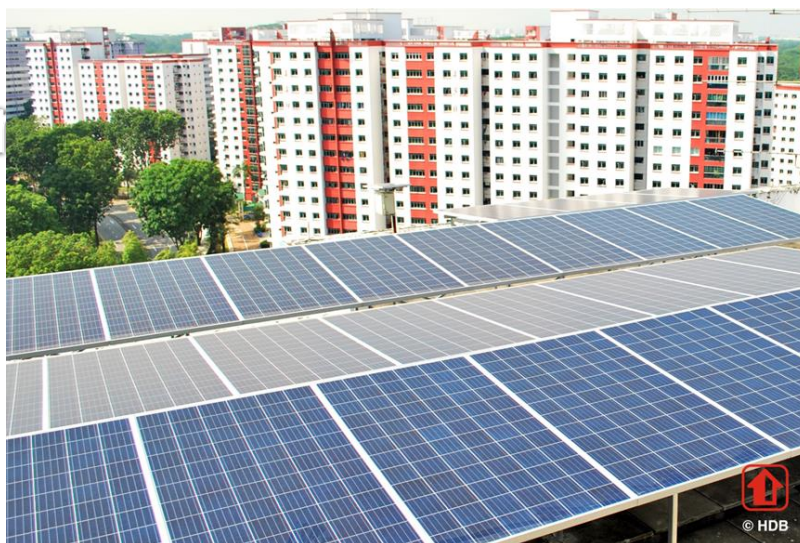
By 2020, more than half of the existing 10,000 HDB blocks will be fitted with or identified for solar installation
