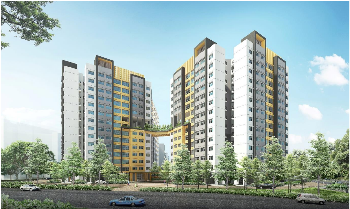
Valley Spring @ Yishun, launched in August 2016, is a pilot HDB project using the PPVC method.
