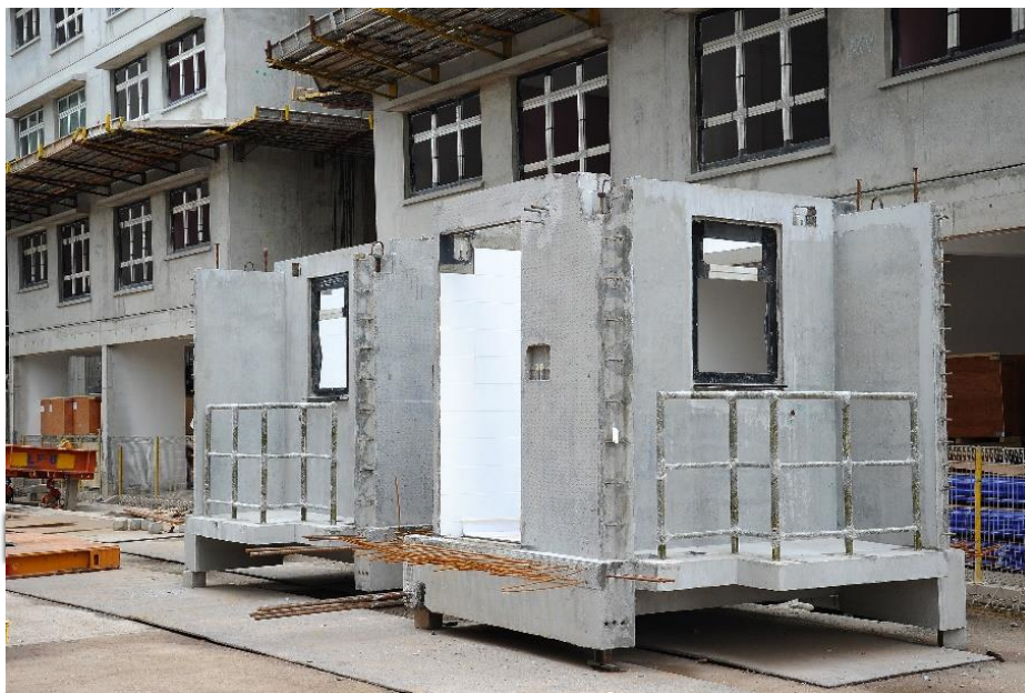
Prefabricated Bathroom Units delivered for installation at the construction site
