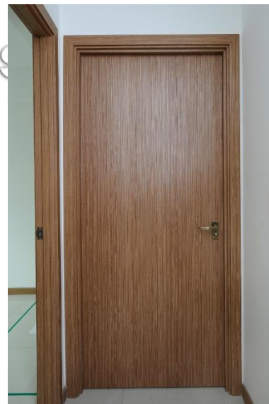
(From left) The vinyl strip flooring and laminated uPVC door and architrave are examples of new materials which HDB has adopted to improve productivity.
