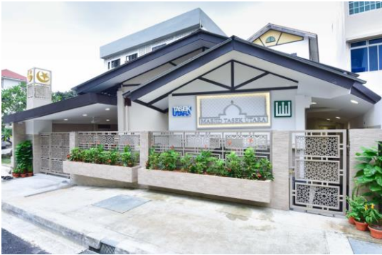
A fresh new look for the exterior facade of Masjid Tasek Utara.
