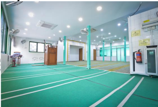
Refurbished main prayer hall of Masjid Hussein Sulaiman.
