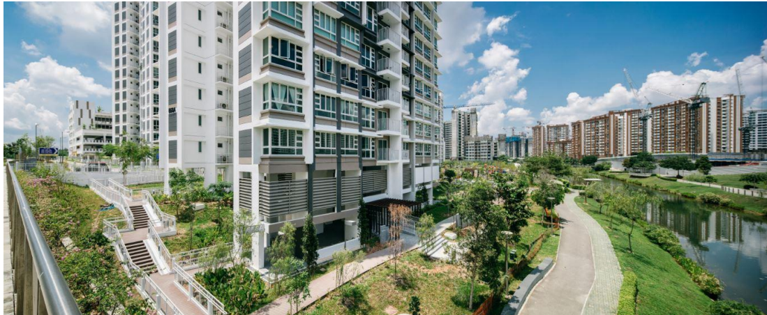
Waterway Ridges is the first public housing development with a large-scale integration of Active, Beautiful, Clean Waters (ABC Waters) elements [Photo credit: Surbana Jurong Consultants Pte Ltd]
