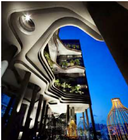
PARKROYAL ON PICKERING: VIEW FROM 5 TH FLOOR LOOKING UP TO UNDERSIDE OF SCULPTED SKY TERRACES
